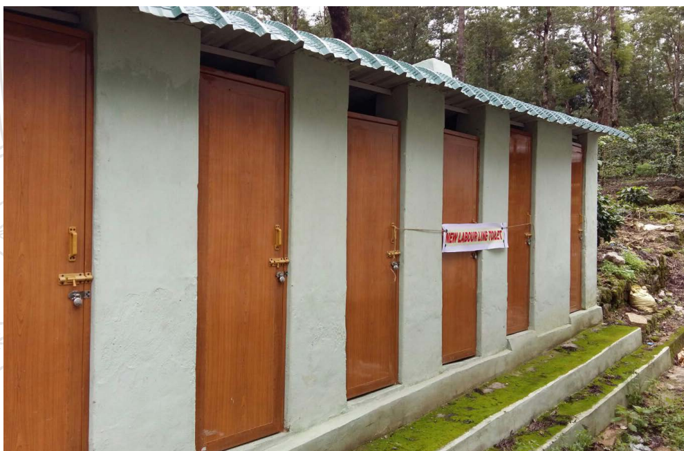
Sanitation blocks at Thalanar Estate - India
